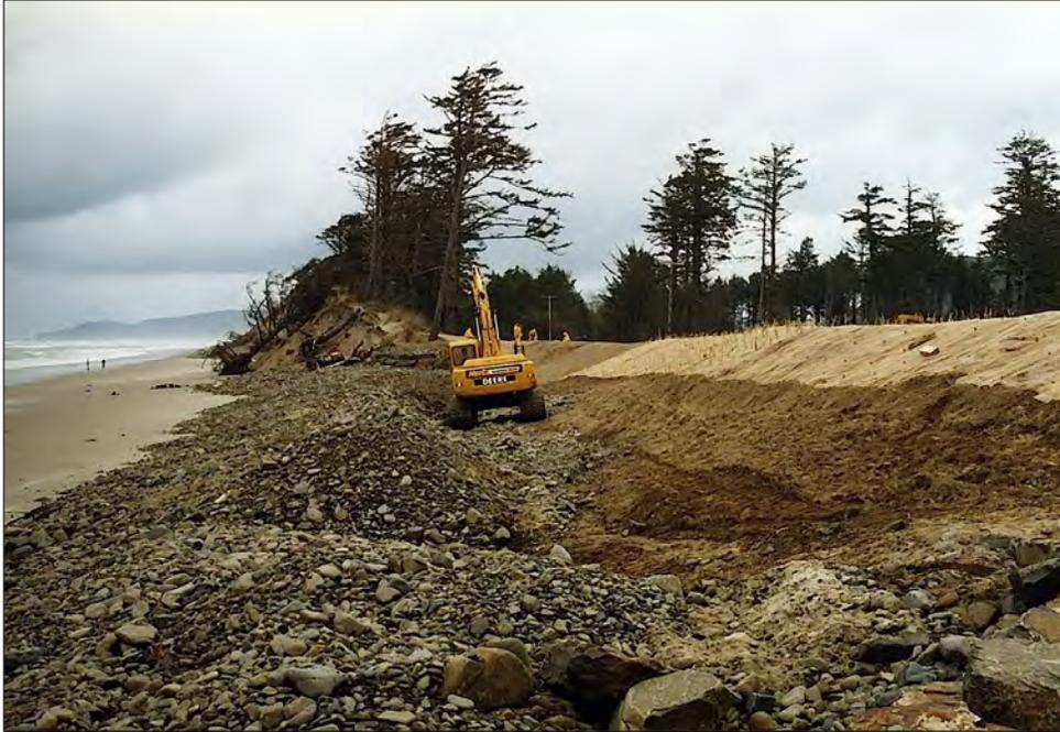
**Figure 6.** Construction of the cobble berm and artificial foredune in Cape Lookout State Park during the fall of 2000. A continuation of the old dune ridge is seen in the background, which had previously extended past this area of erosion.
